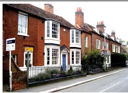
Little Dene, Cottage, Clifton House, High St
