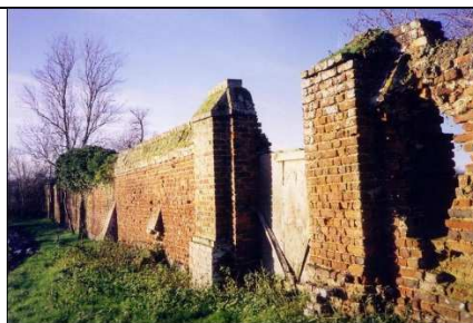
Garden walls, Southlea Farm
